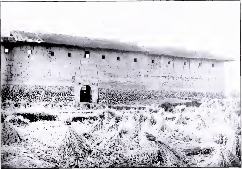
FORTIFIED DWELLING : YUNGCHUN VALLEY (Exterior).
